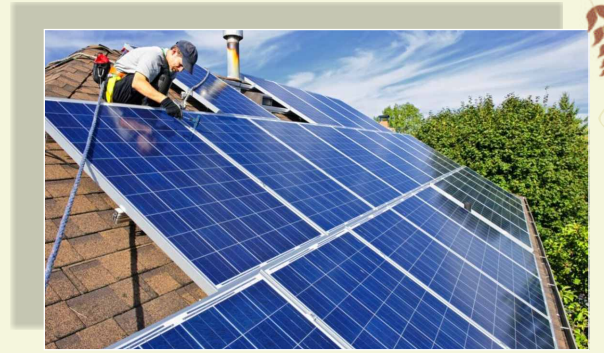
Common Electric Solar
